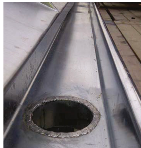
Downpipe outlet starter soldered to gutter
